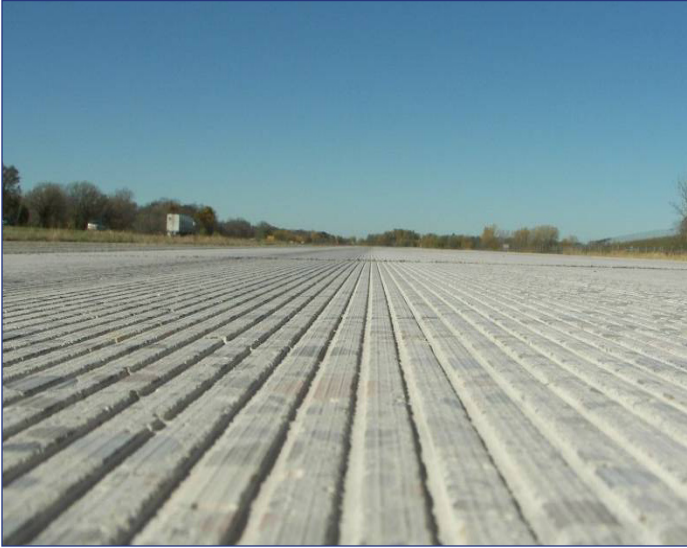
Figure 11. Quiet, longitudinally grooved concrete pavement (photo courtesy of Diamond Surface, Inc.)
