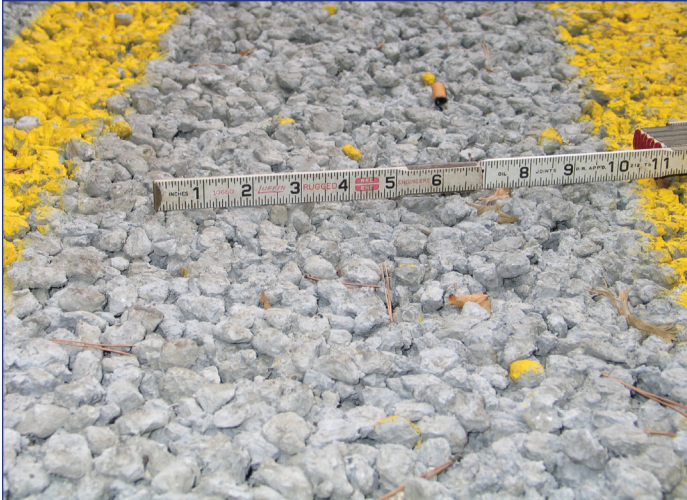
Figure 10. Pervious concrete pavement parking area in Normal, Illinois
