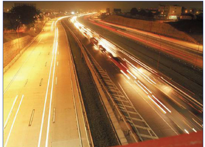
Figure 5. Brazil roadway illustrating concrete (left) vs. asphalt albedo
